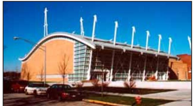
*This campus landmark features a cable-stayed system that suspends S-shaped roofs over large-volume gymnasium and natatorium spaces.*
