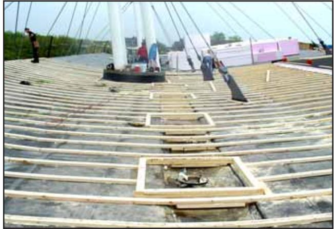
*This massive construction project required 2,000 tons of steel alone, featuring 120-foot-tall steel masts that support approximately 2 million pounds of roof.*
